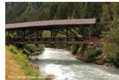
Foto: Tobias Haase wooden footbridge CC BY 2.0
